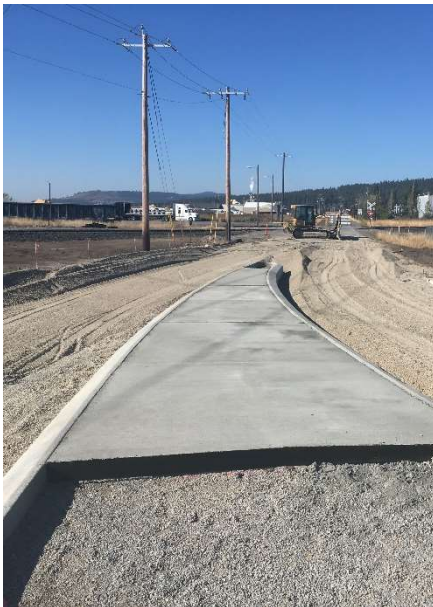
Concrete is Nearly Completed
