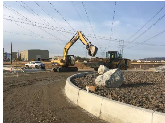
Roundabout Curbs are in and the Road is Ready for Paving
